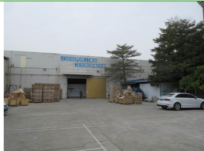
Factory workshop building view
