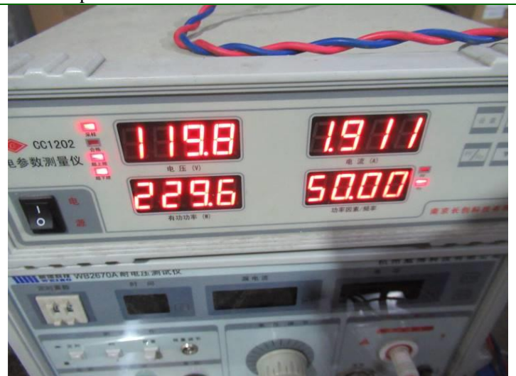
162. Power Consumption Check
